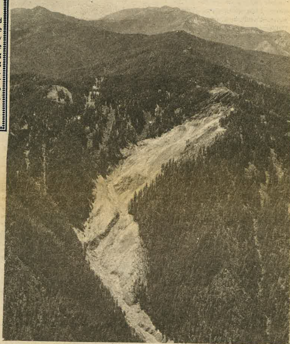
Road-triggered landslide, Smith River watershed
