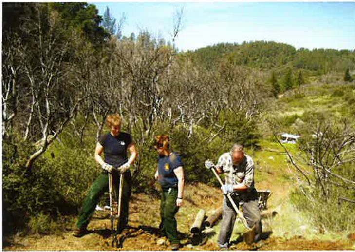
Digging post holes — PHOTO: SARAH STEELE WILSON
