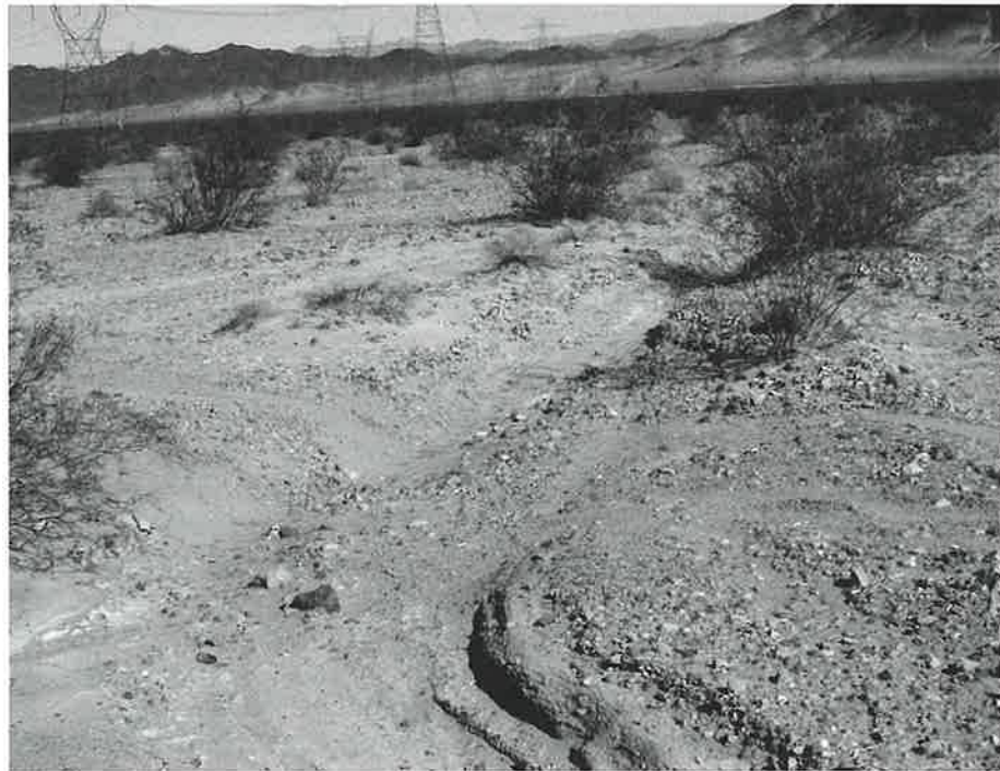
Bogus highways: a washout and deteriorated track in the Soda Mountains...
