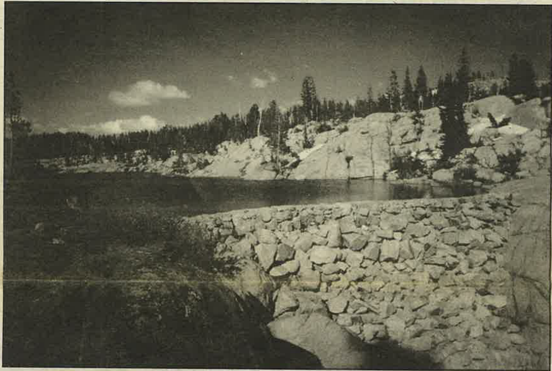
Y-Meadow Dam in the Emigrant Wilderness. This dam is 25 feet high and creates a totally artificial lake. Later, as the lake is drawn down mudflats and a bathtub ring become evident. Photo by Steve Brougher.
