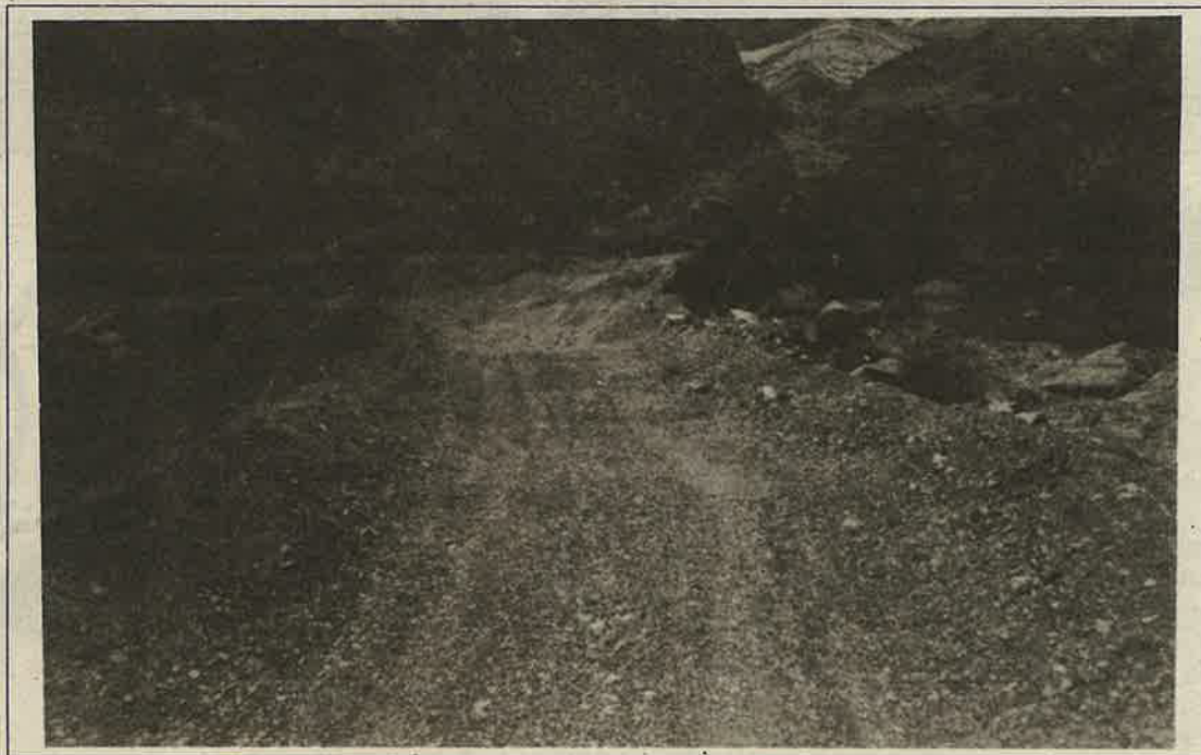
After: The narrows (from a greater distance). The Bureau of Land Management intervened before a miner could finish bulldozing a road through the narrows to his Saline Valley mineral claim.
